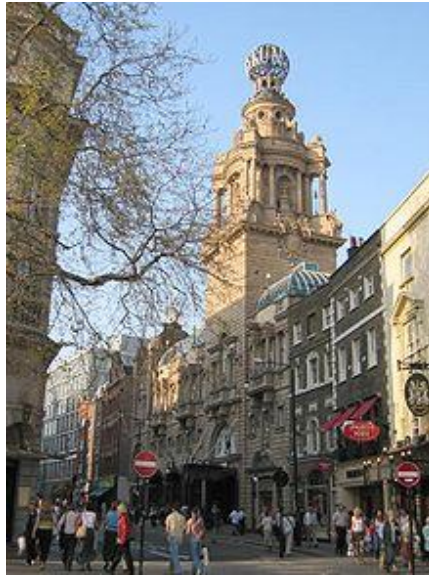
A recent photograph of the 1904 London Coliseum, one of many Frank Matcham-designed theatres with London's widest proscenium arch.
